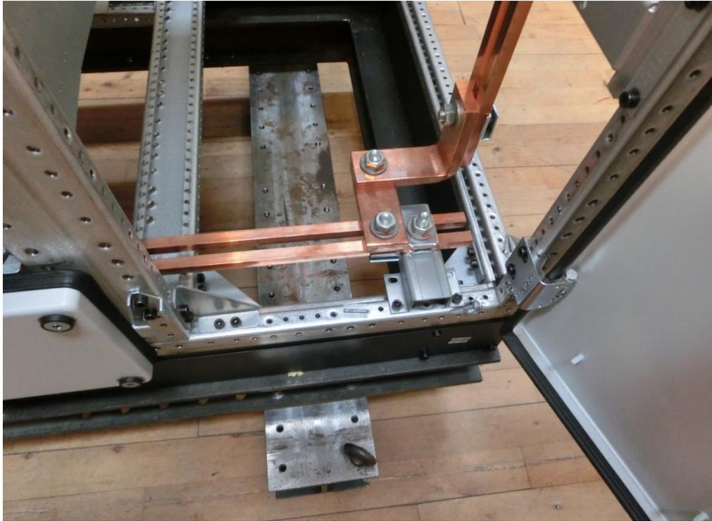
Photo 25 Visual Inspection: Large copper bars and mounting OK.
