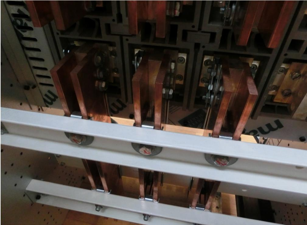
Photo 19 Visual Inspection: Large copper bars and mounting OK.
