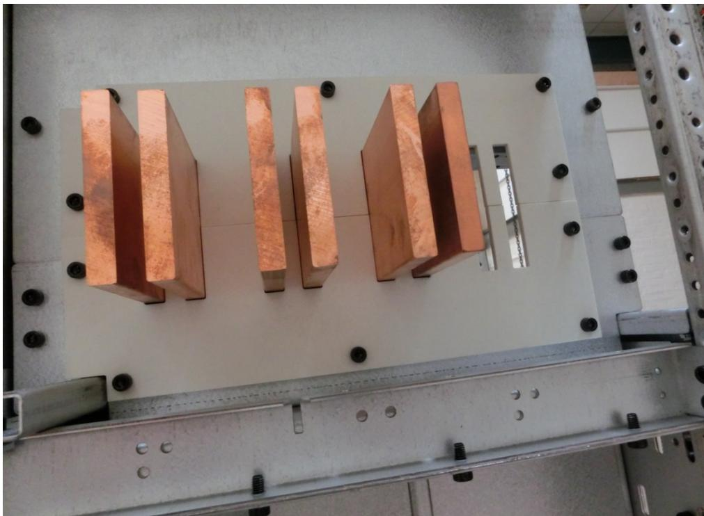
Photo 26 Visual Inspection: Large copper bars and mounting OK.
