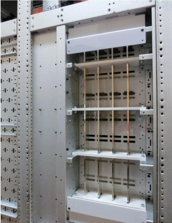
Photo 30 Visual Inspection: Medium size cupper bars and mounting OK.
