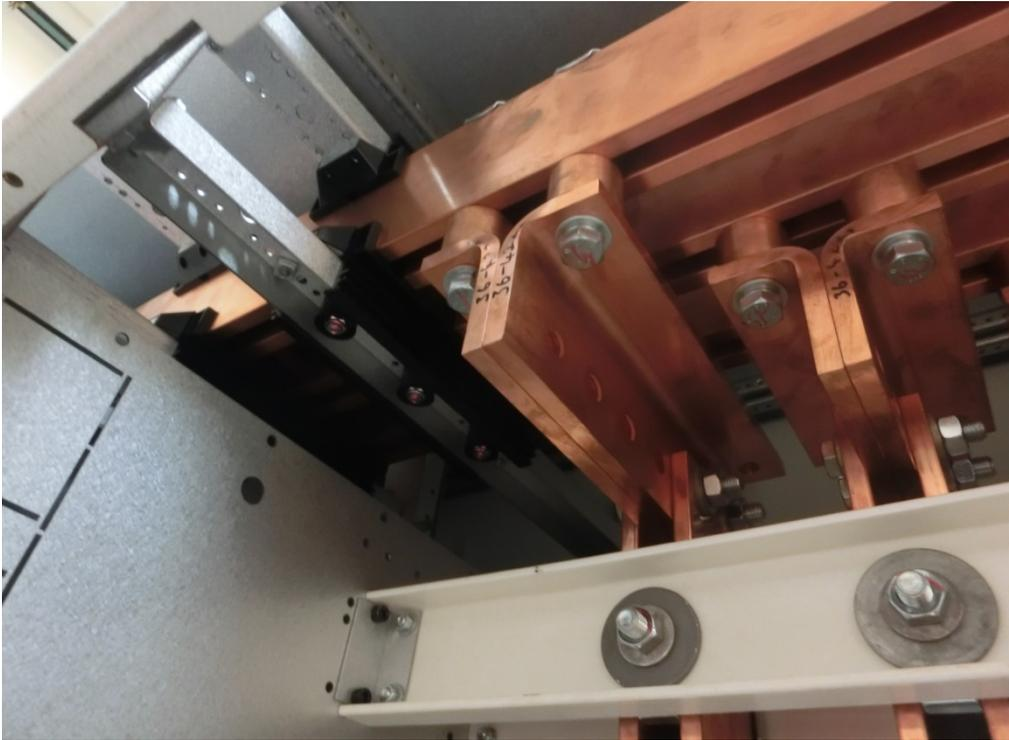
Photo 21 Visual Inspection: Large copper bars and mounting OK.
