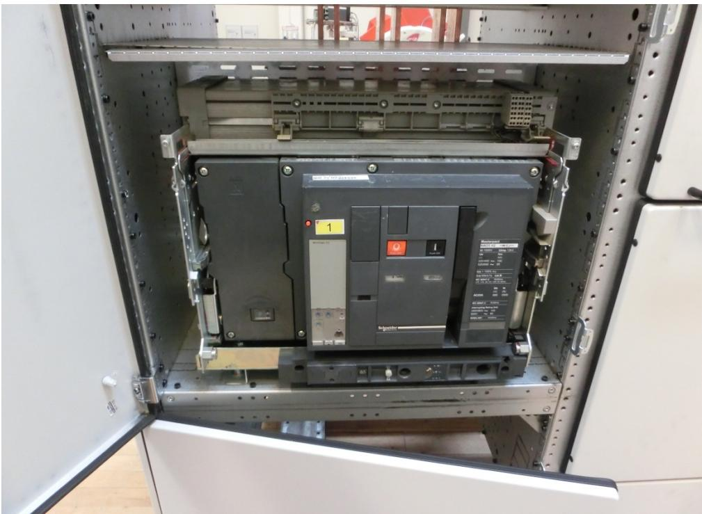
Photo 22 Visual Inspection: Large circuit breaker and mounting OK.
