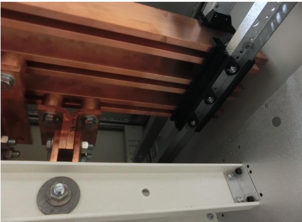
Photo 20 Visual Inspection: Large copper bars and mounting OK.
