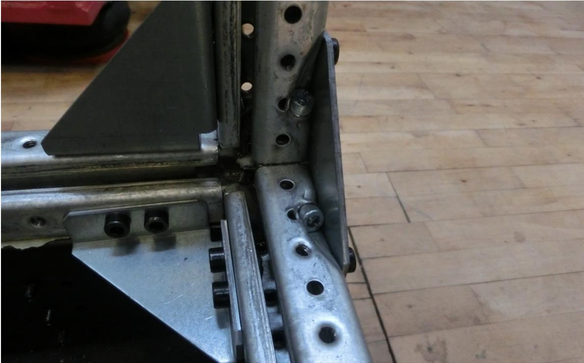
Photo 29 Visual Inspection: "Earthquake brackets" OK.
