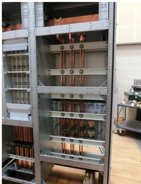
Photo 18 Visual Inspection: Large copper bars and mounting OK.
