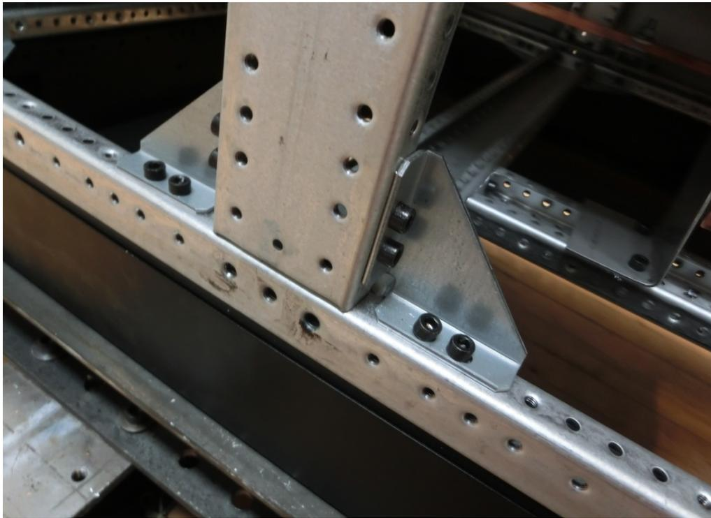
Photo 27 Visual Inspection: “Earthquake brackets” OK.
