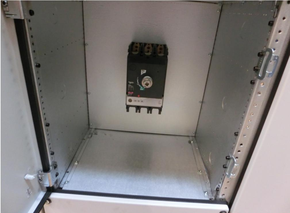
Photo 23 Visual Inspection: Small circuit breaker and mounting OK.
