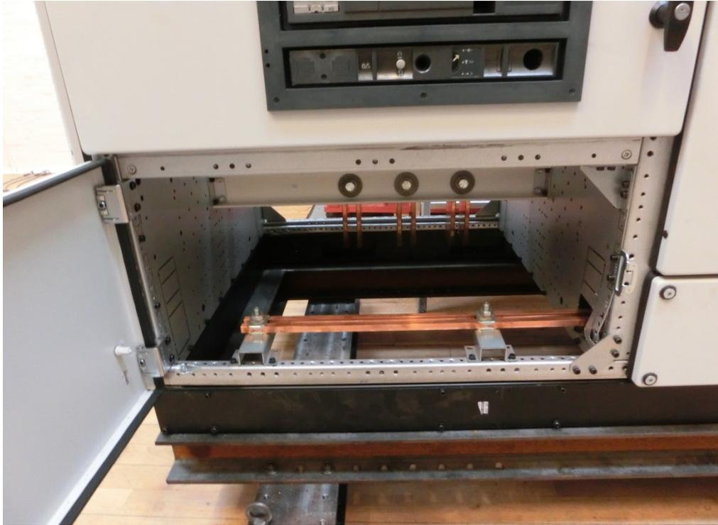
Photo 15 Visual Inspection: Large copper bars and mounting OK.
