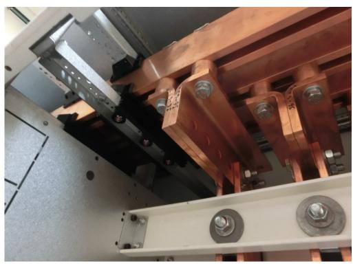
Photo 21 Visual Inspection: Large cupper bars and mounting OK.
