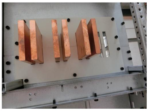
Photo 26 Visual Inspection: Large cupper bars and mounting OK.
