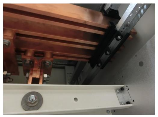
Photo 20 Visual Inspection: Large cupper bars and mounting OK.
