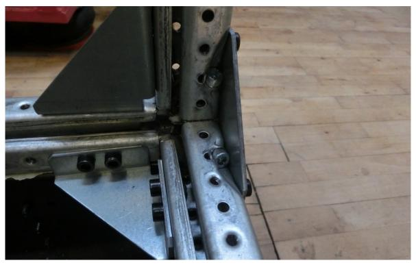
Photo 29 Visual Inspection: "Earthquake brackets" OK.
