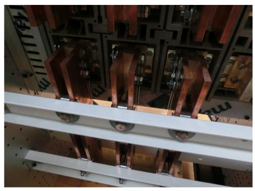
Photo 19 Visual Inspection: Large cupper bars and mounting OK.
