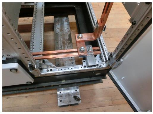
Photo 25 Visual Inspection: Large cupper bars and mounting OK.
