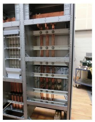
Photo 18 Visual Inspection: Large cupper bars and mounting OK.
