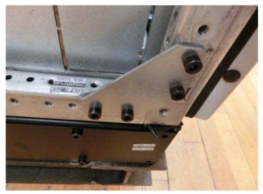
Photo 28 Visual Inspection: "Earthquake brackets" OK (black frame broken).
