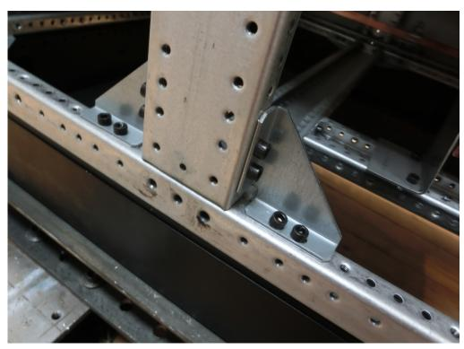
Photo 27 Visual Inspection: "Earthquake brackets" OK.
