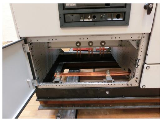
Photo 15 Visual Inspection: Large cupper bars and mounting OK.
